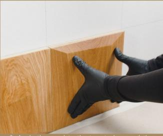
3. Apply the panel to the target place, and then press it over the entire surface so that the glue is evenly connected to the substrate.
